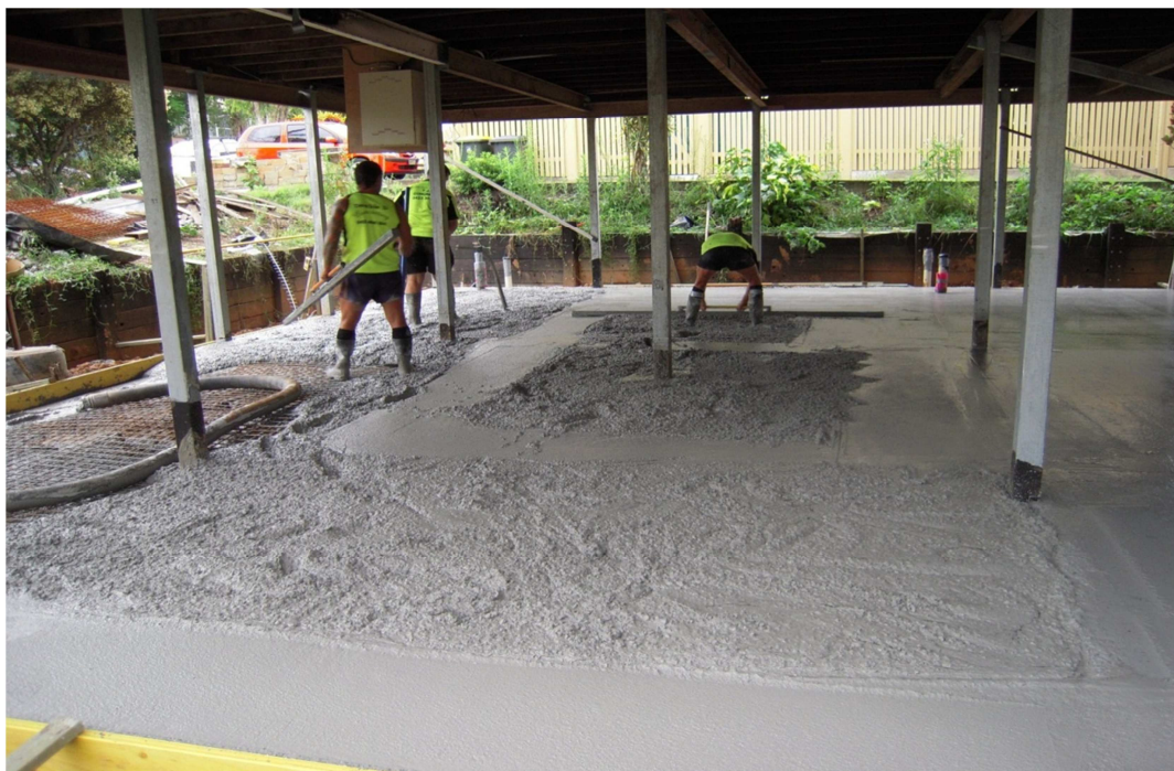
Figure 7 - Bill Ennals Brisbane 32MPa (Nominal) Pour. Note the Warm Margarine Like Rheology
