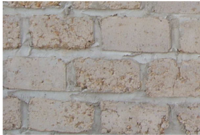
Figure 1 – Eco-Cement Mud Bricks and Mortar
