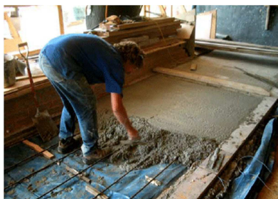
Figure 2 – Eco-Cement Floor using locally dug chalk as Aggregate
